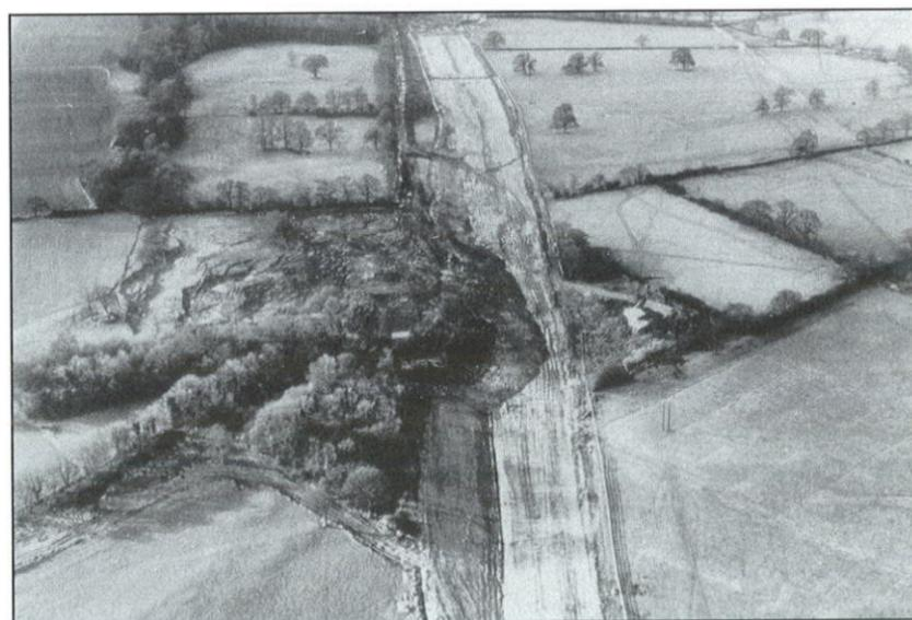
Fig. 9: Landslides into the cutting for the M4 motorway (during construction), near Swindon.
