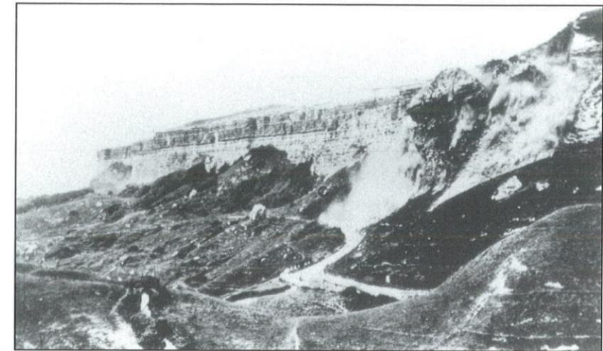
Fig. 25: The toppling failure of 1928 at Gore Cliff, Isle of Wight, in mid-air (acknowledgements to Dr. A. N. INSOLE, Sandown Museum, Isle of Wight).
