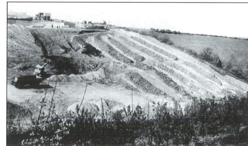
Fig. 32: Trench and counterfort drains under construction at Boulby, Yorkshire (acknowledgements to Imperial Chemical Industries Ltd., Agricultural Division, and to Cleveland Potash Ltd.).
