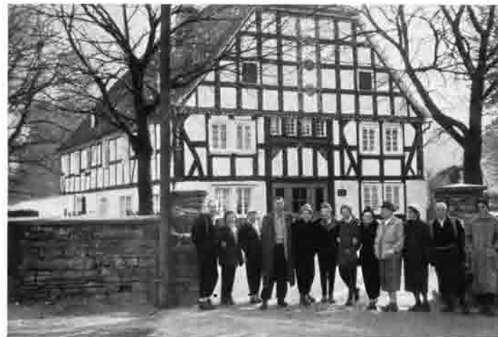
In Saalhausen — Lennetal
