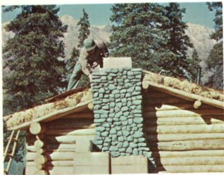
A collapsible form speeded the work.
