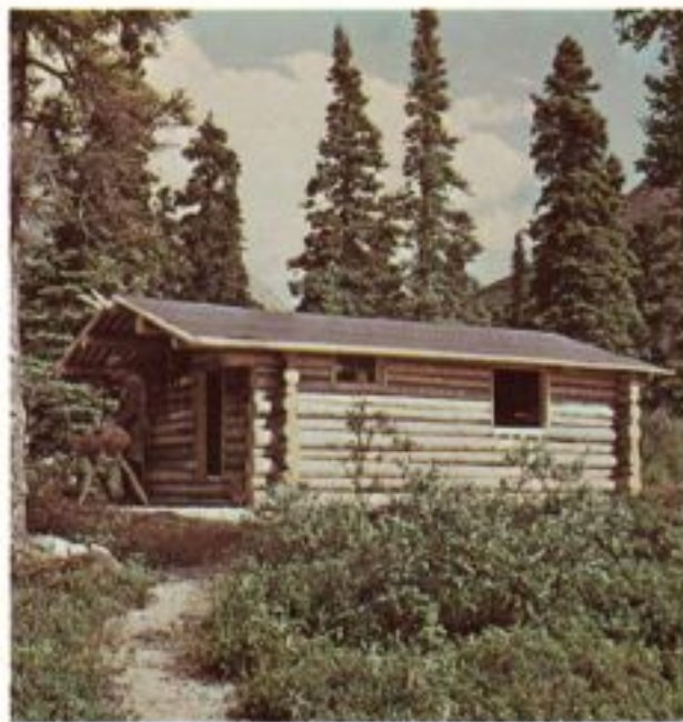
The cabin looked better with a tar-paper roof.
