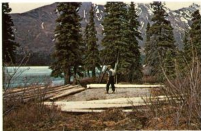
Side logs were bedded on a floor of gravel.
