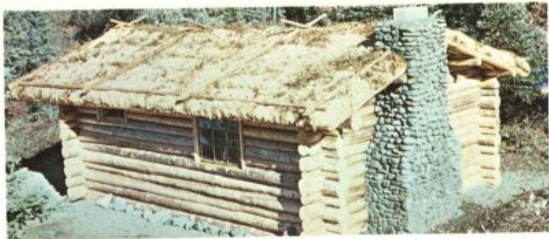
The fireplace was about ready for a test.
