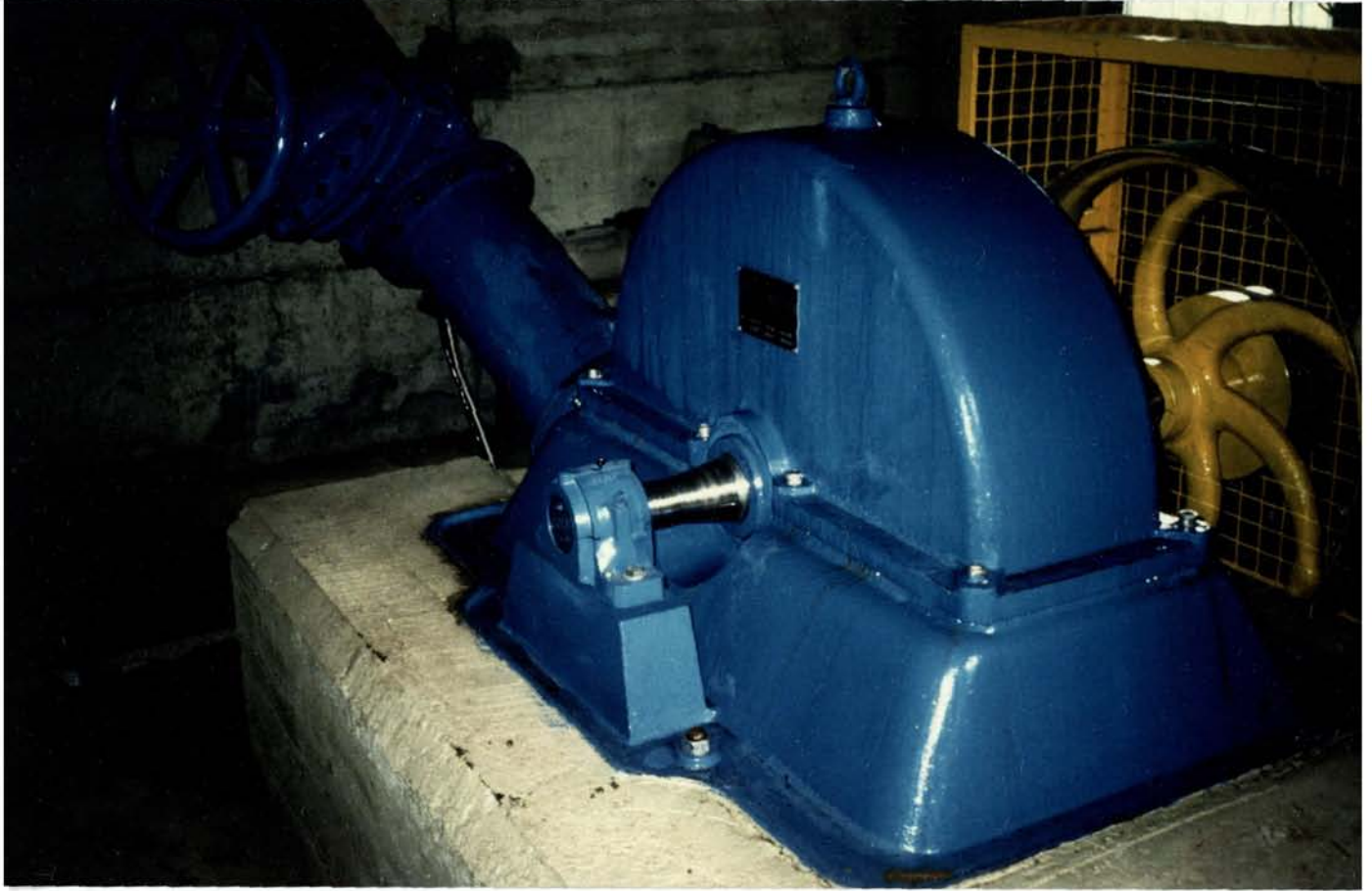
Pelton-turbine, eindüs. Fabr.: Fa. Geppert, Baujahr 1991, QA = 150 l/s, nT = 330 min -1 , NT = 48,0 kW
