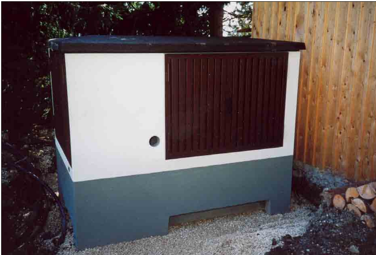
20 kV-Kabelstation Brunnstein
