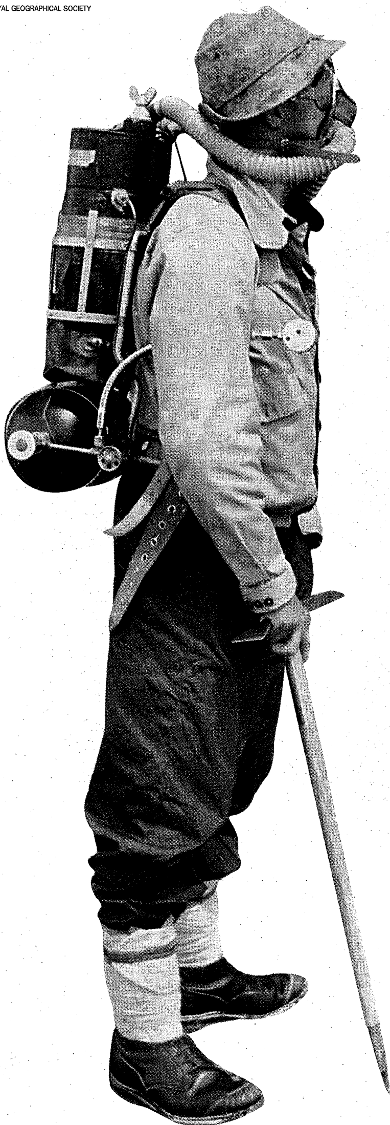
An early version of the oxygen cylinder, some of which weighed 47lb
