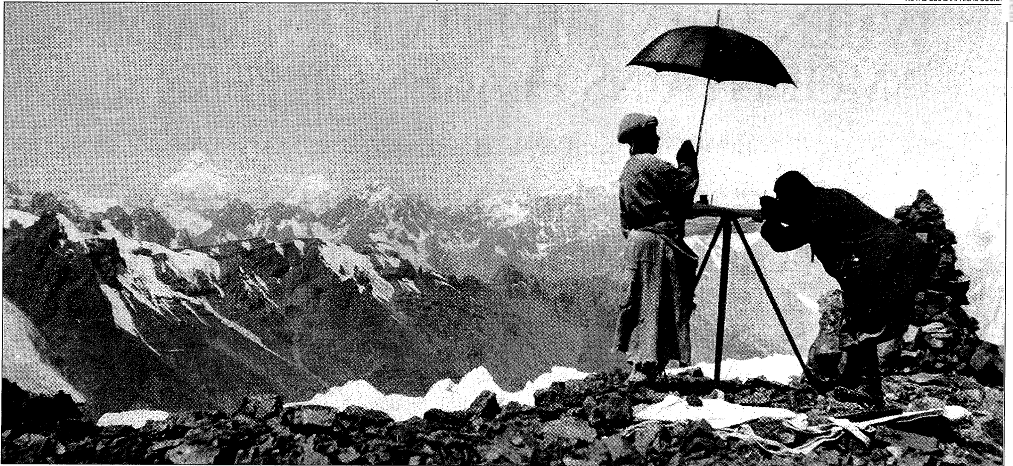
As British rule spread across the plains of northern India, surveyors followed in its wake. Here, Khan Sahib and Afraz Sul Khan are plane tabling from the Tartar La in Kashmir
